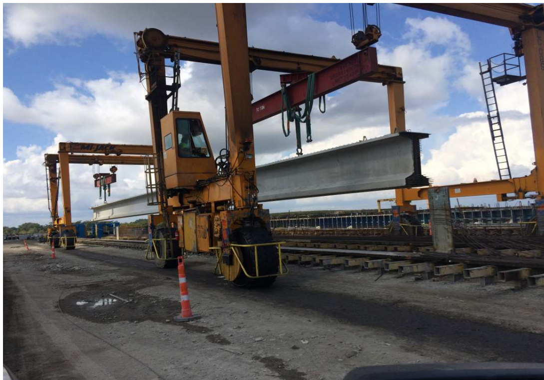
Figure 2. Typical prestressed bridge beam being fabricated at Valley Prestressed Products
