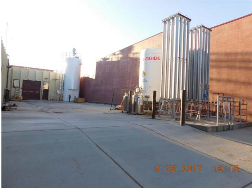
Figure 3. Liquid Nitrogen Storage tanks installed above underground bulk storage tanks.
